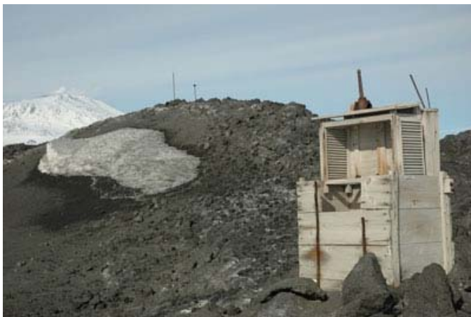
The 100-year-old Steven's box at Cape Royds with Mt Erebus in the background. Thermometers were inside and an anemometer spun on the metal spoke sticking upwards from the top. The door long ago blew away; it had slats as well. A person had to open the door, read the dials and then record the data in a notebook.
